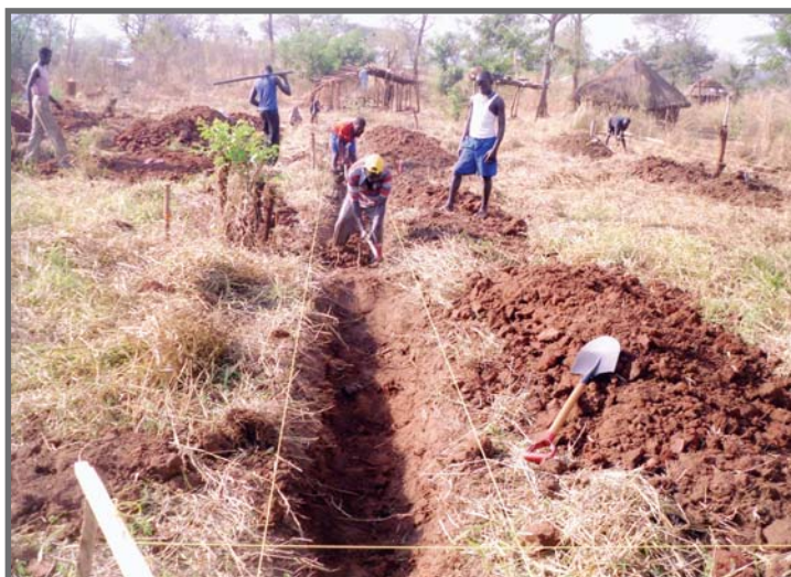
Workers digging trenches for the foundation of a building on campus.
