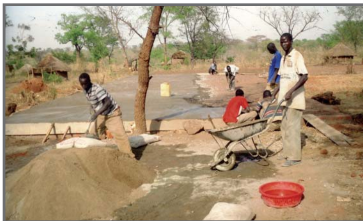
Mixing the sand, gravel and cement for the building foundation.
