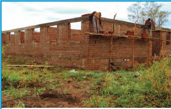
Finished walls of the preacher training school building
